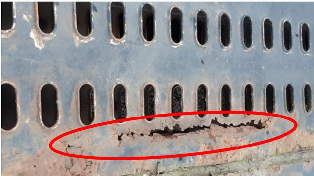
Figure 1A: oxidation passing through the decking
